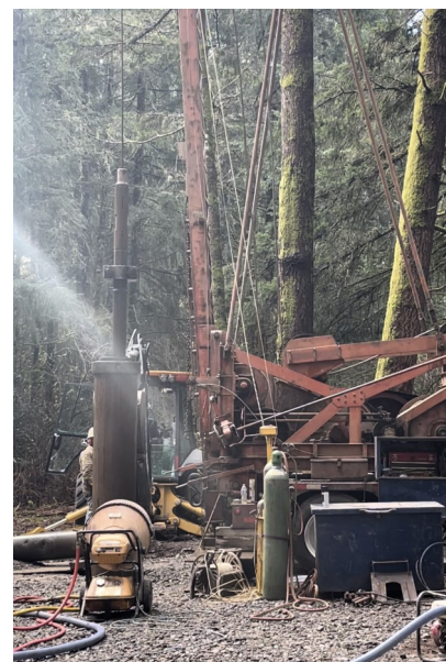
The new Casebolt well being drilled.
